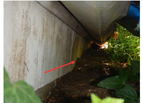
Lower walls at ground
