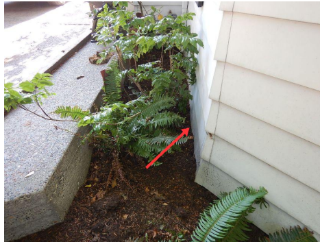
Lower walls at ground
