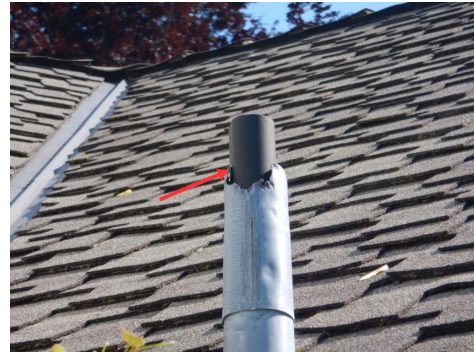
Damaged flashing
