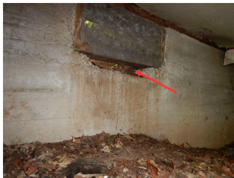
Damaged vents
