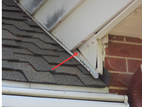
Improper transitions
