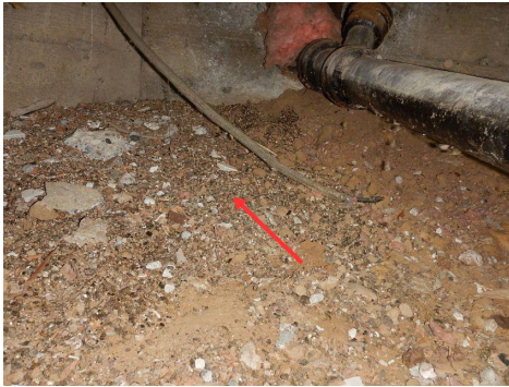
Vermiculite in crawlspace
