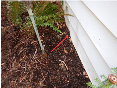
Lower walls at ground
