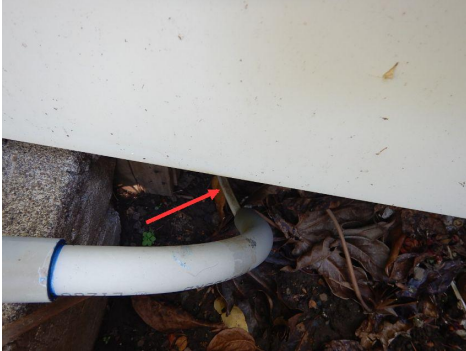
Improper wiring
