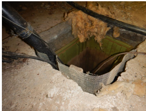
Drain in crawlspace
