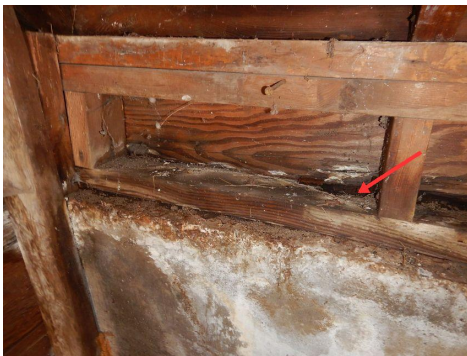
Rot and insect damage
