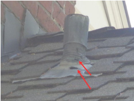
Damaged flashing
